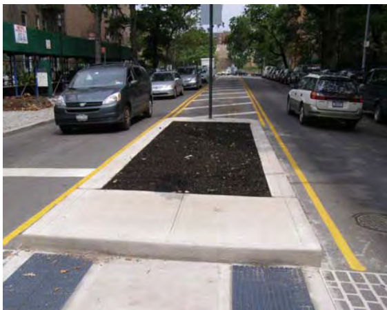
Planted Median Refuge with Roadway Narrowing
