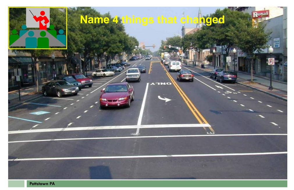
Fewer travel lanes; added bike lanes; parallel to back-in diagonal parking on one side; new pavement
