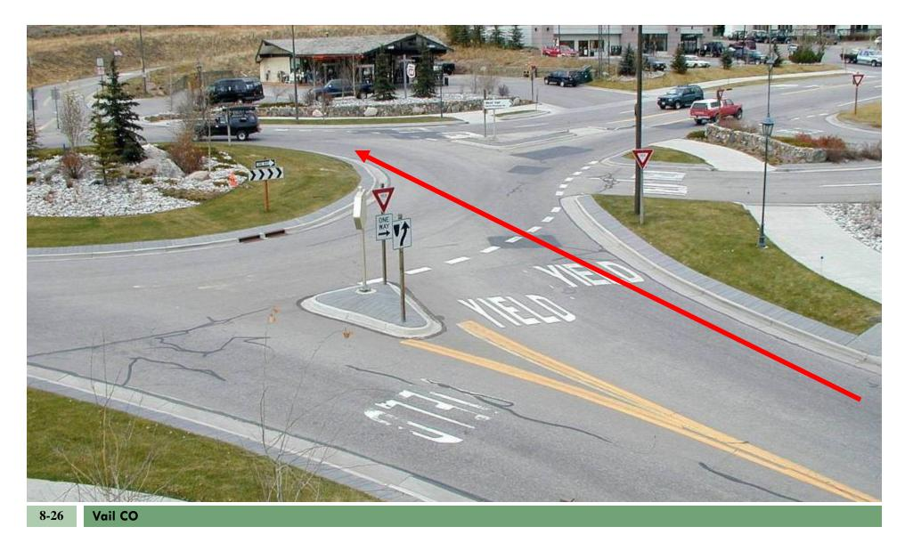
Drivers may take a straighter, faster path on entry and exit, resulting in higher speeds – lane markings are recommended to minimize this
