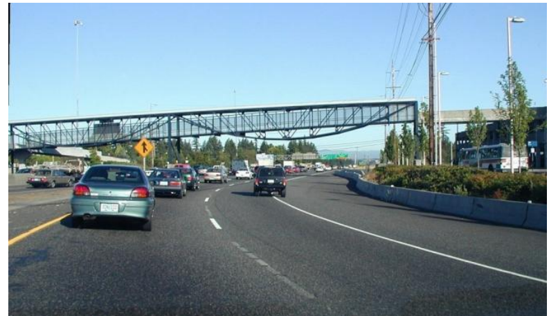
Light rail stations
